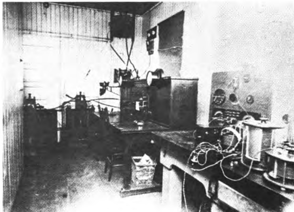
KFS - SAN FRANCISCO BEACH STATION - 1910 The station was equipped with a 12-KW Arc. at this time. It was placed in operation July 1910 with the original 12 KW Danish Arc. Two 300' masts were constructed as towers for the facility.
